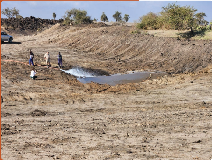
Desilting and Strengthening the Dams at Maanzoni Conservation Area
